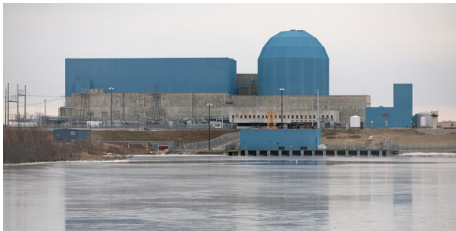
Clinton nuclear plant
