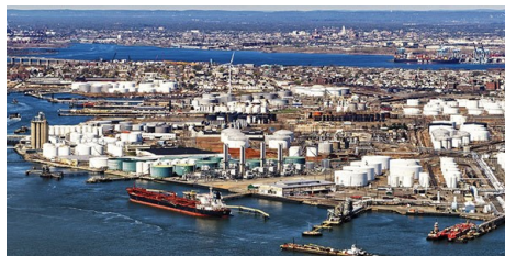
Bayonne Energy Center | Direct Energy
